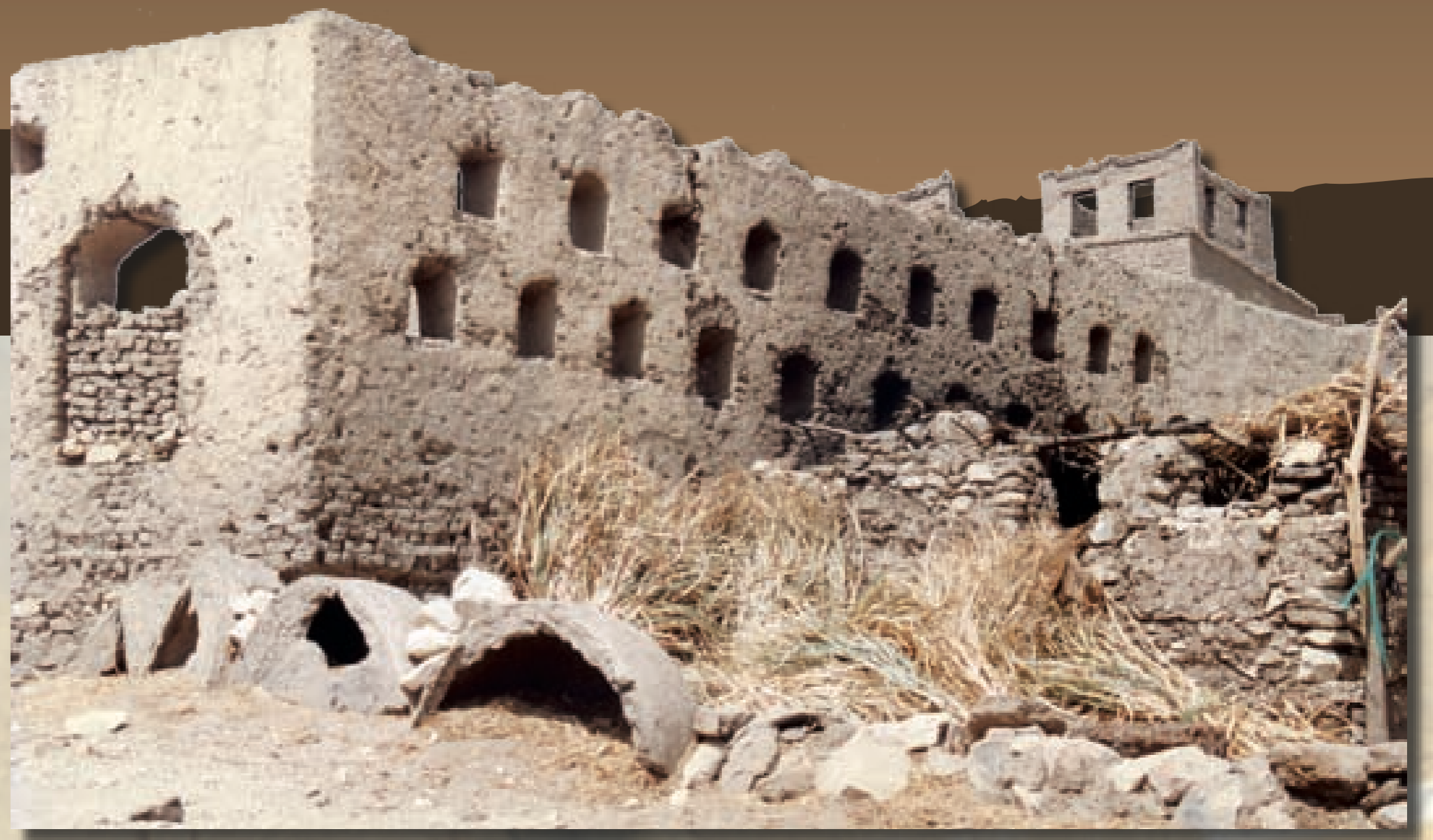
Kitchen and zawyeh deserted long ago. The wood is stripped out of the houses when people move - to be used again or sold.
